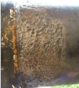
Fig. 5. An outer defect found in a seamless gas pipeline. OD = 16", nominal WT = 10 mm, length: 250 mm, width: 450 mm, metal loss: 58%.
