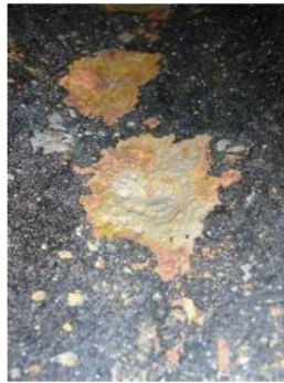
Fig. 6. An inner defect in a seamless crude oil pipeline. OD = 6", nominal WT = 4.8 mm, length: 56 mm, width: 48 mm, metal loss: 52 %
